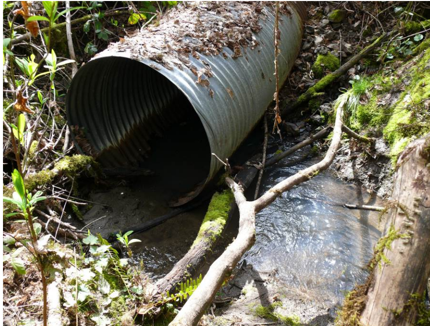
Figure 6: Upstream view of the Richards Creek culvert which crosses below the road at the south end of the main stem restoration area. This is a barrier to fish migration because the downstream side is perched above the stream
