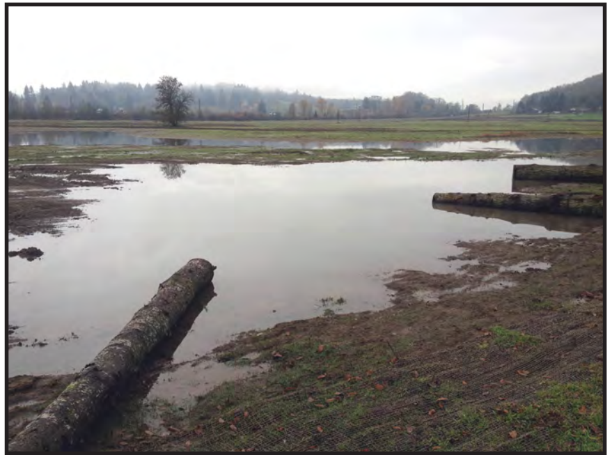
Wood placed in recently constructed vernal pool
