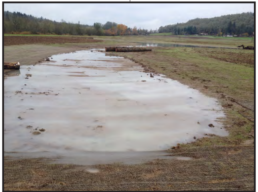
An agricultural ditch can be re-contoured into a broad, shallow swale as shown above, adding hydrologic diversity to a site (shown prior to planting).
