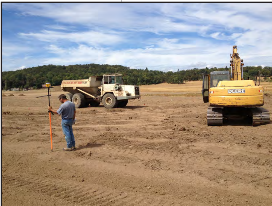
Re-grading a smoothed agricultural field during site preparation to create topographic variation and vernal pools conditions
