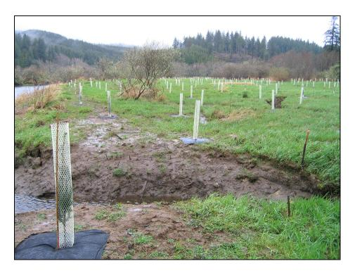
Photo A6. March 17, 2008: Site S65 north-facing view of dike breach and former pasture; partial dike removal and extensive shrub and tree plantings can be seen (white Vexar tubes). Photo by Laura Brophy.
