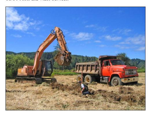
Photo A3. August 14, 2007: Excavation of pilot channel at site S65. Jeffrey Jones measures channel depth while Nathan Large operates the excavator. Photo by Laura Brophy.
