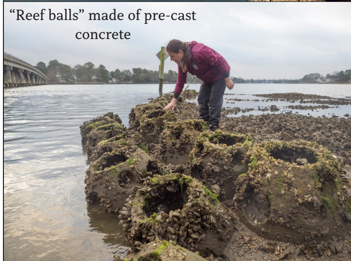
Oyster reef made of pre-cast concrete rings
