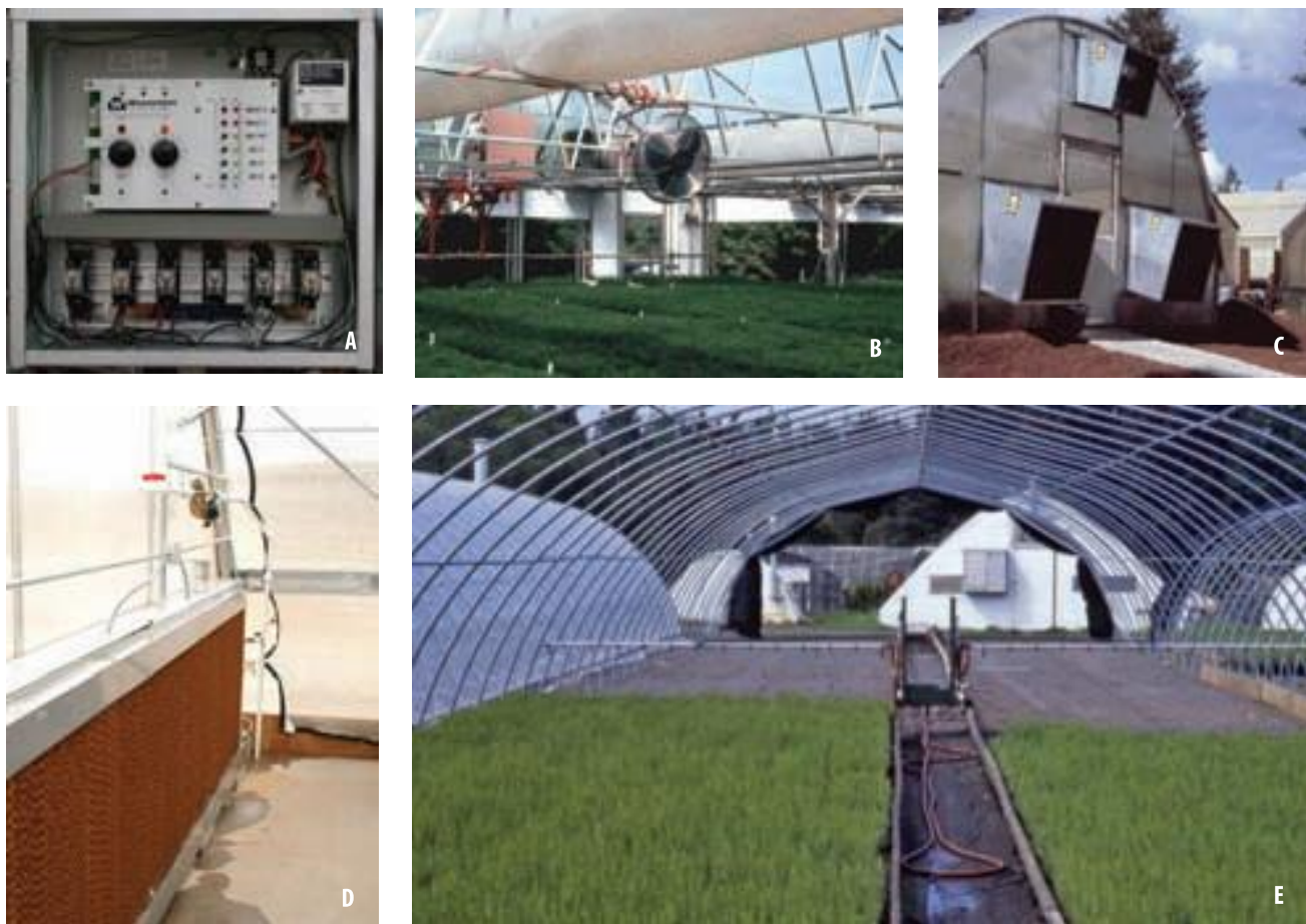
Figure 4.15 —(A) Fully controlled greenhouses contain heating and cooling systems and sophisticated controllers. (B) Greenhouses heat up quickly during sunny weather and must be designed for cooling with interior circulation fans and (C) exhaust fans and vents. (D) In dry climates, fans pull air through wet walls, where it is cooled by evaporation. (E) A quick application of irrigation water can also be used to cool crops. Photo A by Jeremy R. Pinto, B-E by Thomas D. Landis.
