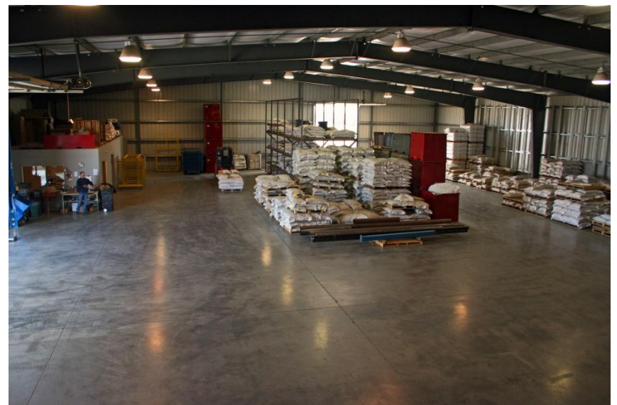
Seed storage warehouse
