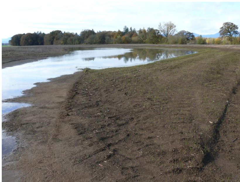
Figure 15. Flooded swale in and recently constructed berm in prairie site preparation area, October 2016.
