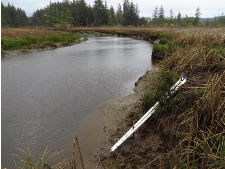
Fig. 11. Channel water level and salinity logger installation at Cooperage Slough. Two stilling wells are placed side-by-side, one housing a level logger and the other housing a salinity logger. Both loggers are at the same elevation.
